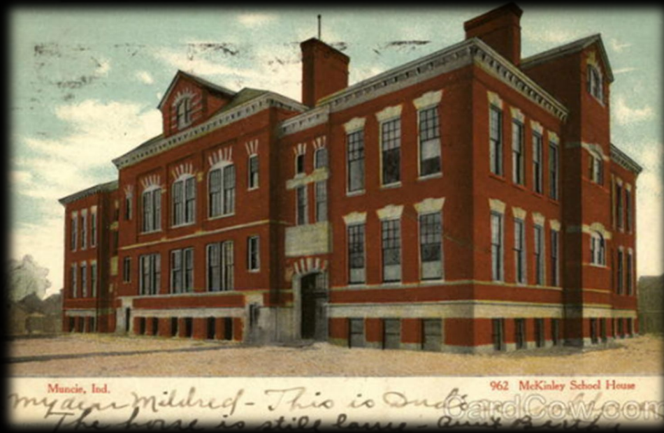
McKinley Elementary School
