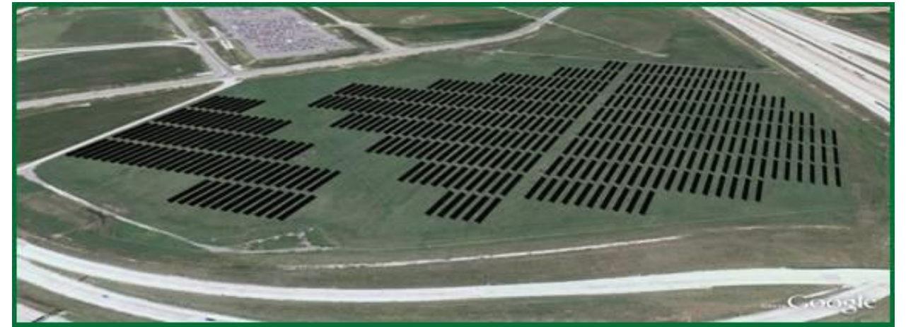
Figure 18: Indianapolis Airport solar farm 37
