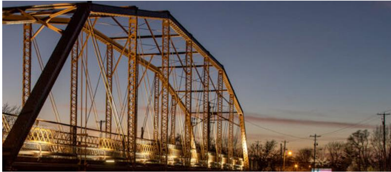
Figure 30: Photograph of the Kitzelman Bridge 55
