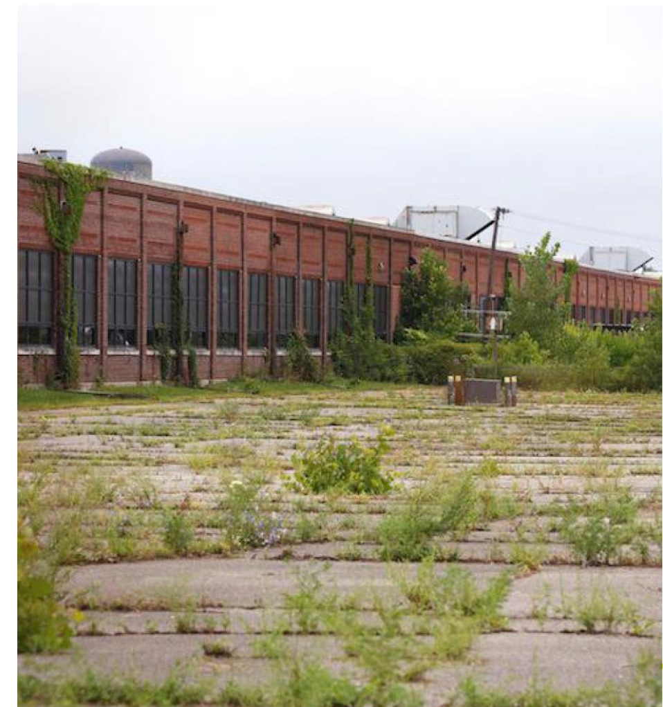
Figure 5: Former Borg Warner Site 13
